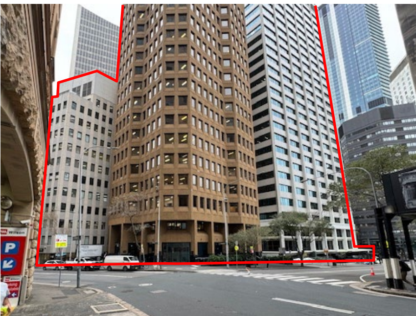
Figure 6. Looking west towards the subject site (in red) from Bent Street
